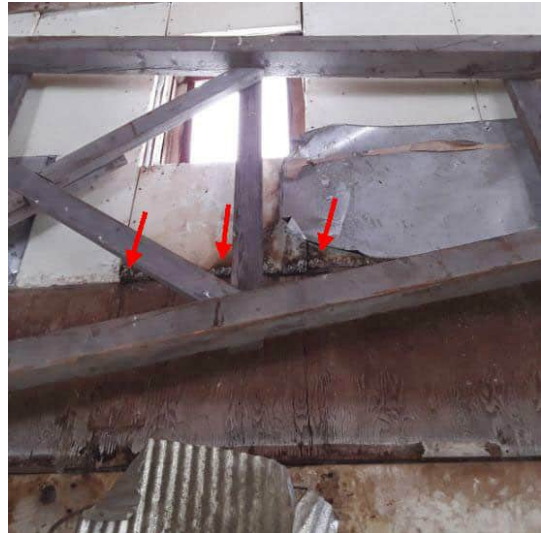
First Floor East Wall B
