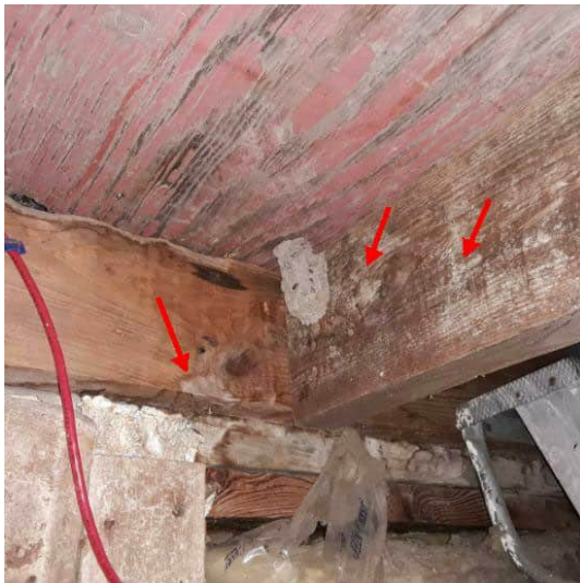
Third Floor West ceiling joists
