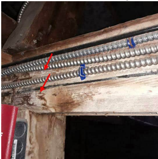
Third Floor West wood beam
