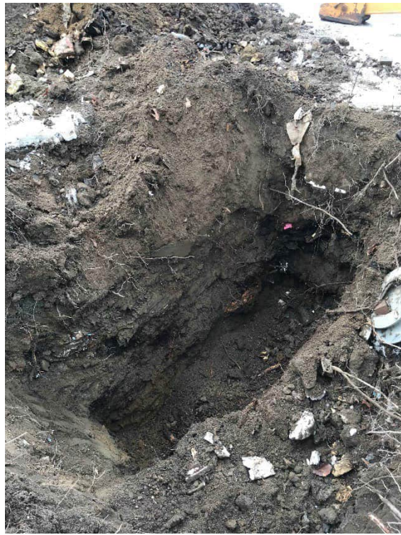
Photo #4: Another view of Test Pit 3 in the “Paint Dump” area on the northern side of the Recycling Barn. Note: waste material buried below grade.
