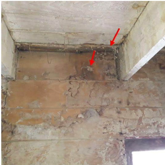
First Floor Center ceiling joists
