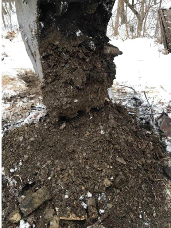
Photo #11: Buried waste material excavated from the "Burn Pit".
