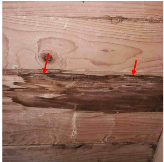
First Floor Center ceiling
