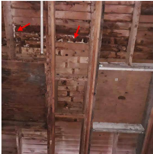
First Floor West ceiling C
