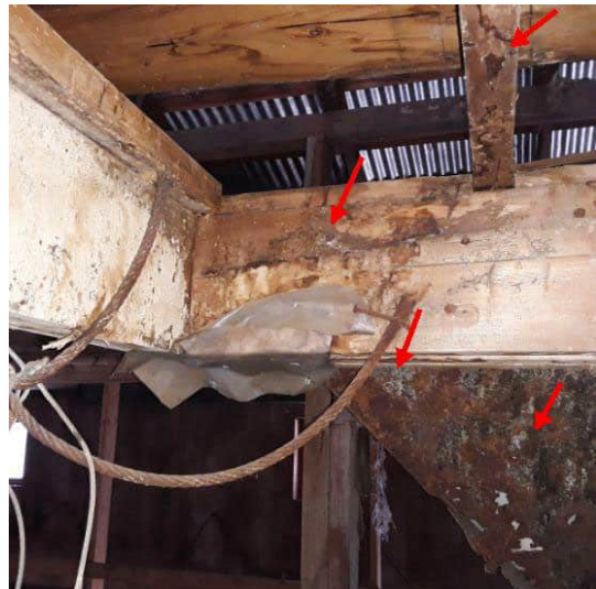
Third Floor East ceiling joists B
