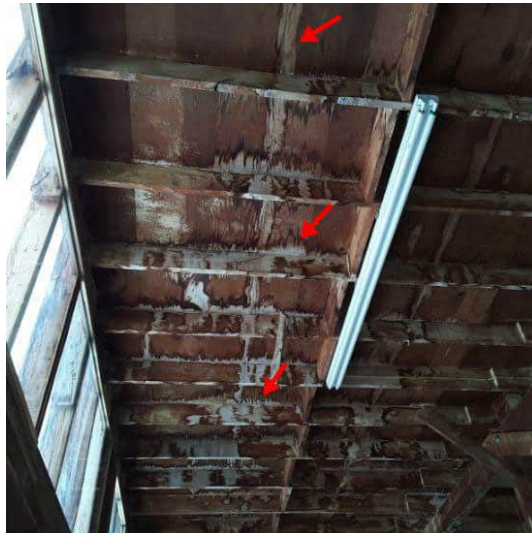
First Floor Center ceiling
