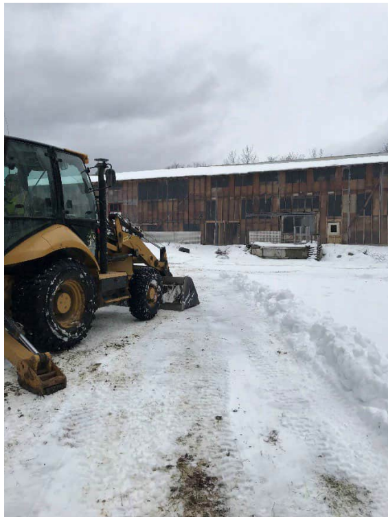
Photo #10: A view of the machine digging in the burn pit, approximately 150 feet south southwest of the loading dock of the Recycling Barn. Note: proposed test pit in “Former Septic Leach Field” to the immediate left of the loading dock. This test pit was not installed at the direction of Town Manager due to concerns that this leach field is actually in use.
