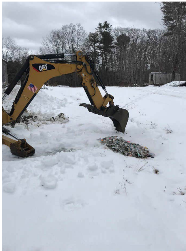
Photo #8: A view of Test Pit 6 at waste glass dumping location facing east.
