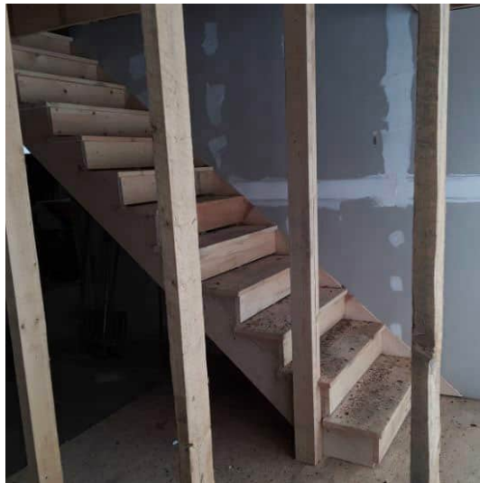
Stairway Control Sample location East
