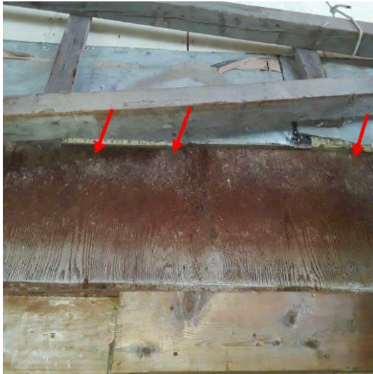
First Floor East Wall A
