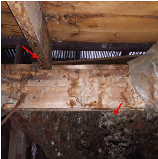
Third Floor East ceiling joists A
