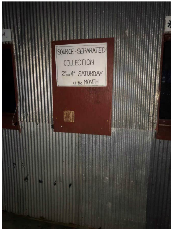
Photo #14: A view of paint sampling location on exterior of building.
