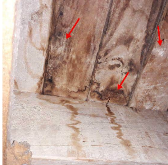
First Floor West ceiling B
