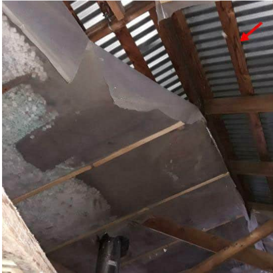
Third Floor West ceiling
