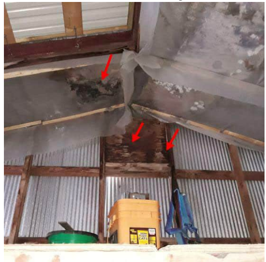
Third Floor West ceiling and wall
