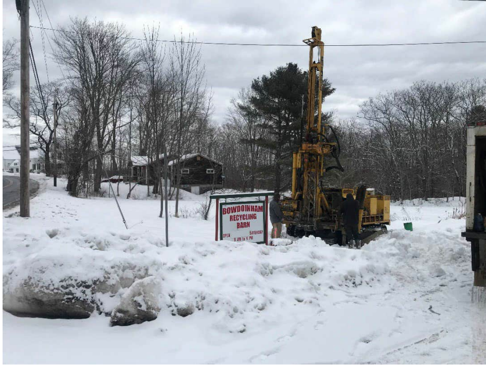
Photo #1: A view of drillers installing upgradient monitoring well along Post Road facing north.
