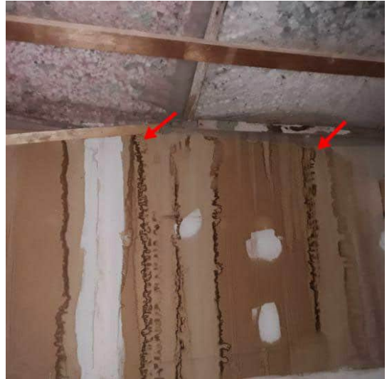
Third Floor West ceiling and wall
