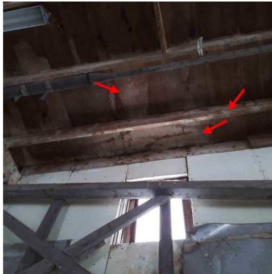
First Floor East Ceiling
