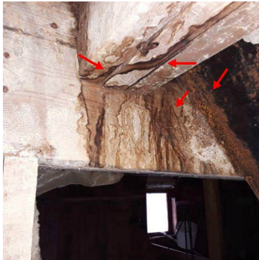
Third Floor East ceiling joists C
