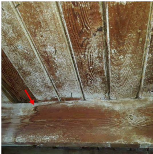
Second Floor West ceiling A
