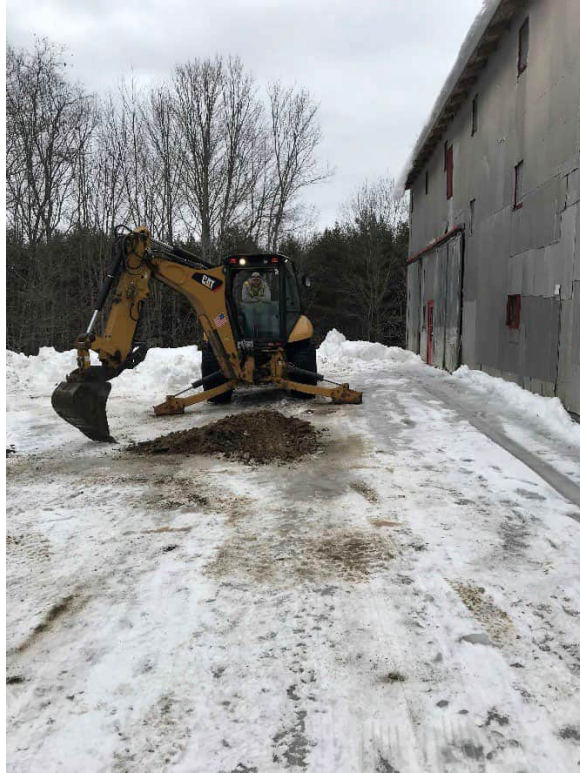
Photo #5: A view of Test Pit 4 in the “Antifreeze Pit” area of the site. Note: the machine was not able to break through densely packed and frozen material to examine this area and collect a sample.
