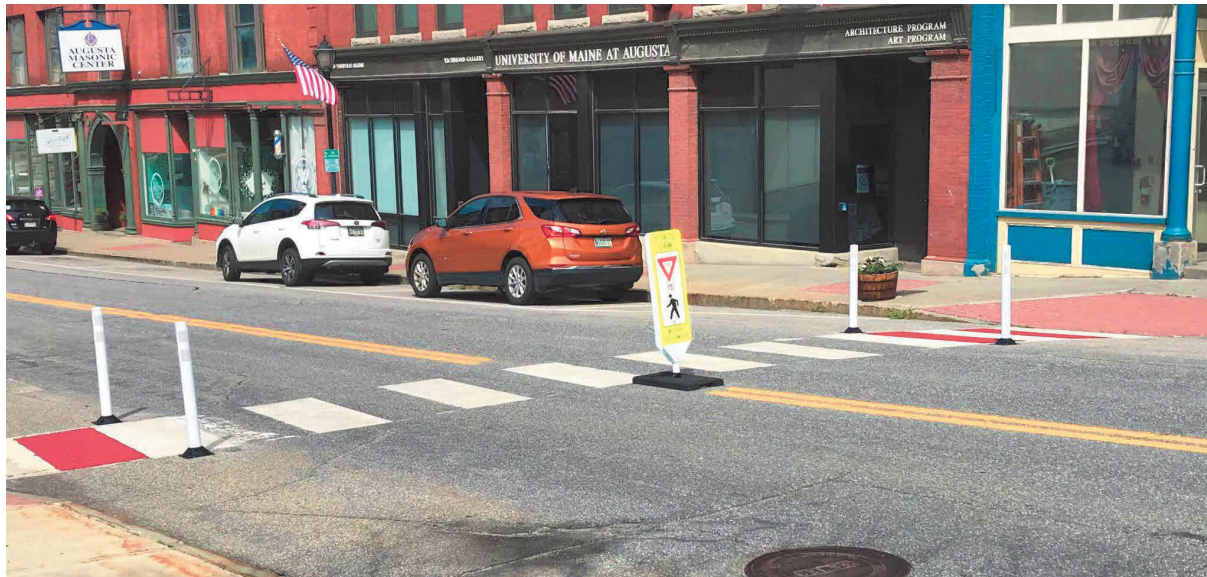
Figure 5. A simple delineator gateway at a crosswalk. R1-6 sign used on center line; a single yellow post may be substituted. Image from Augusta installation 2021
