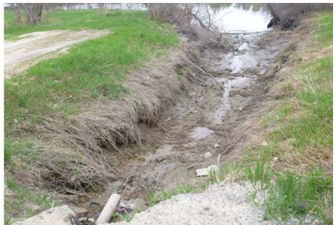
Site Drainage Pipe Outfall & Swale to Cathance River
