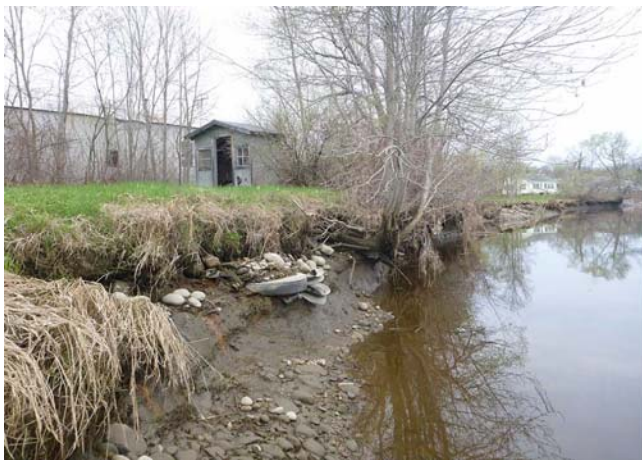
Shoreline behind Public Works Garage Looking North
