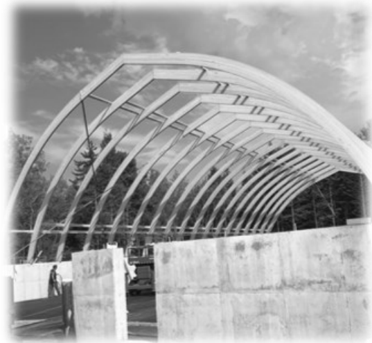
New Salt/Sand Shed at the New Public Works
