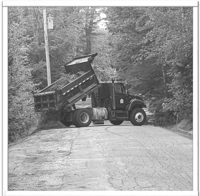
Shoulder Work on Wildes Road
