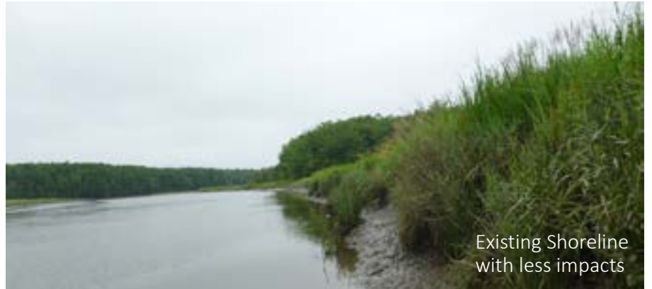
Existing Unstable Shore line and debris
