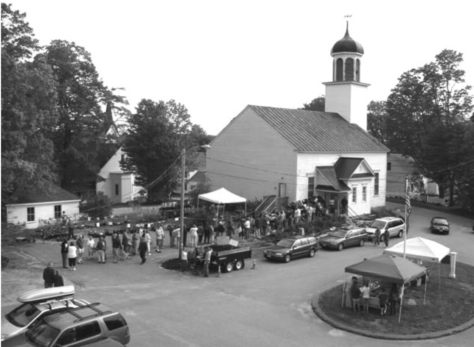
Plant Sale Line after addition of Bathroom in 2000.
