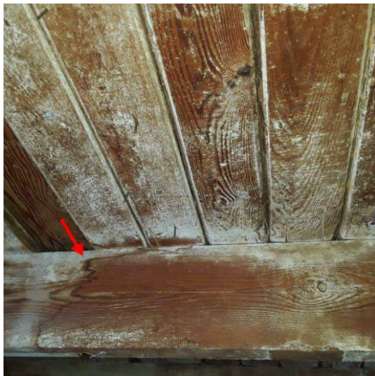
Second Floor West ceiling A
