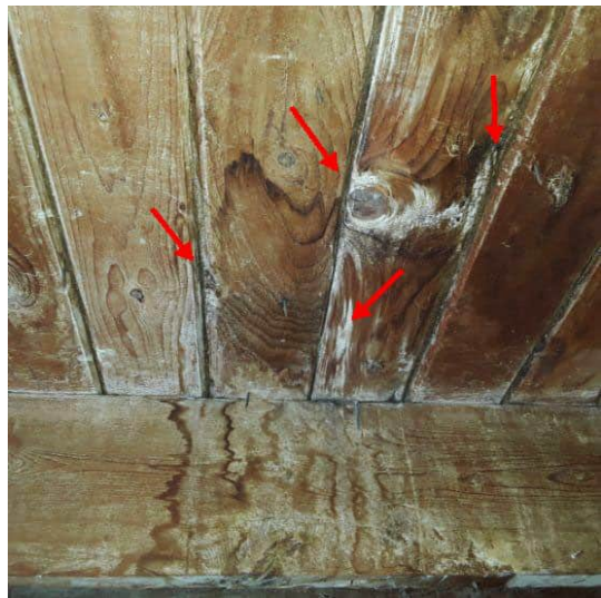
Second Floor West ceiling B
