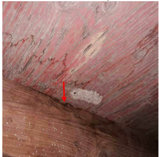
Third Floor West ceiling and wall B
