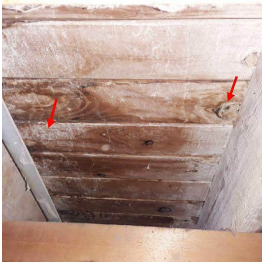
First Floor West ceiling A
