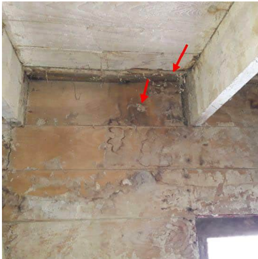
First Floor Center ceiling joists
