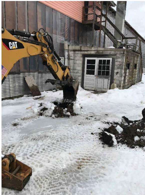
Photo #6: A view of Test Pit 1 (former UST location) on the southern side of the Recycling Barn facing east. Note: boiler located in cinder block room in background.
