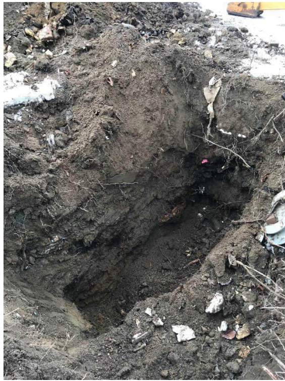
Photo #4: Another view of Test Pit 3 in the “Paint Dump” area on the northern side of the Recycling Barn. Note: waste material buried below grade.
