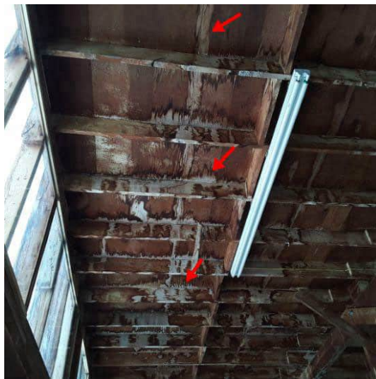
First Floor Center ceiling
