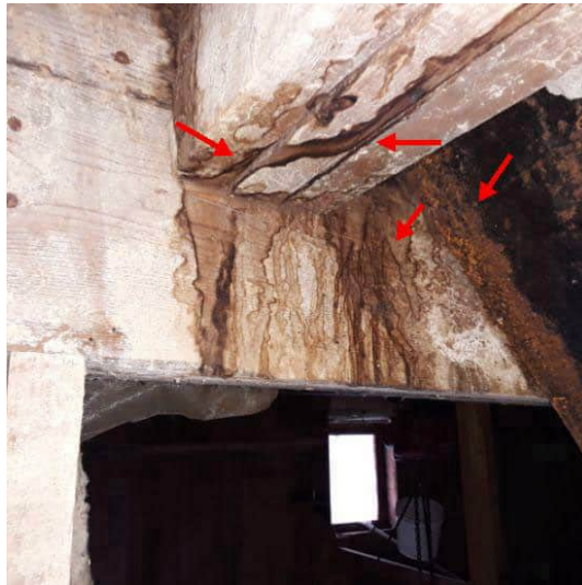
Third Floor East ceiling joists C
