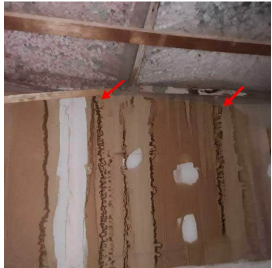
Third Floor West ceiling and wall
