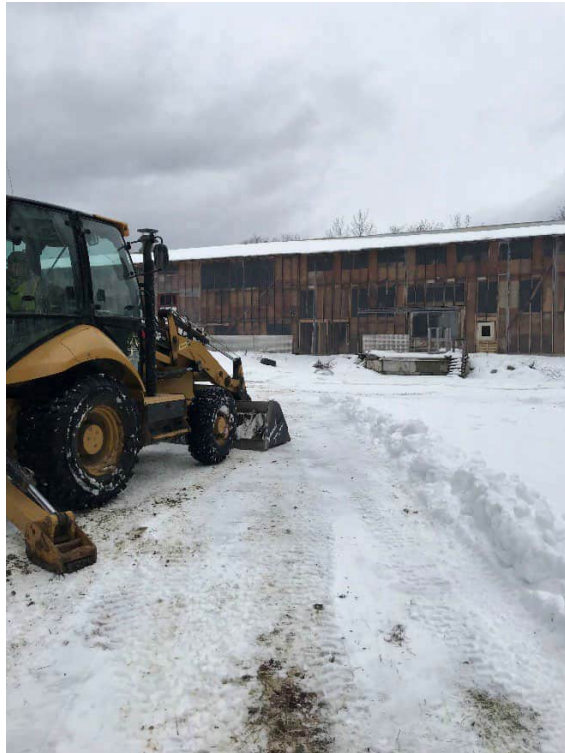
Photo #10: A view of the machine digging in the burn pit, approximately 150 feet south southwest of the loading dock of the Recycling Barn. Note: proposed test pit in “Former Septic Leach Field” to the immediate left of the loading dock. This test pit was not installed at the direction of Town Manager due to concerns that this leach field is actually in use.
