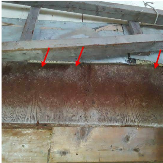
First Floor East Wall A
