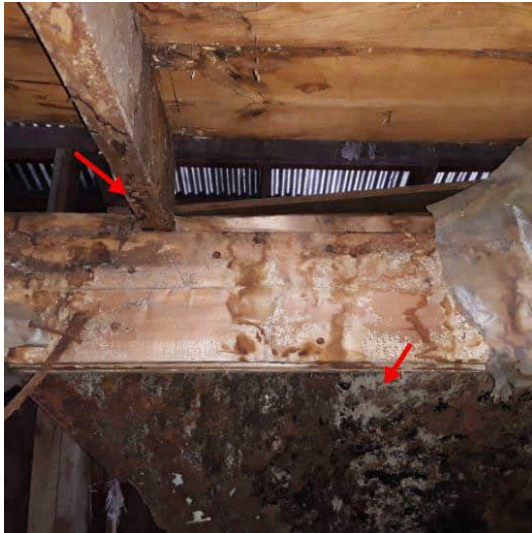
Third Floor East ceiling joists A
