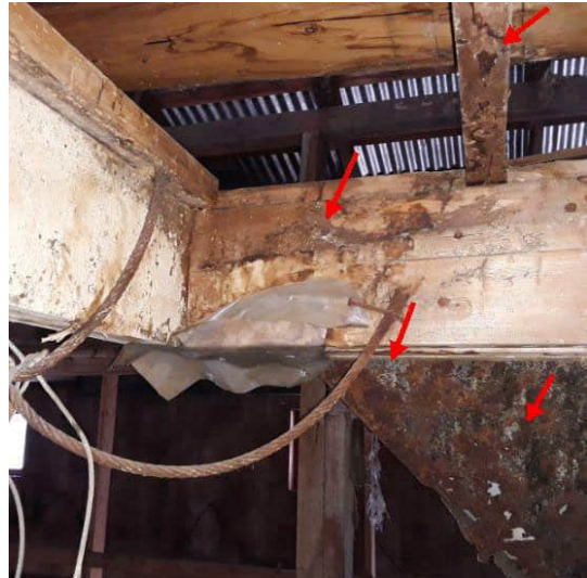
Third Floor East ceiling joists B
