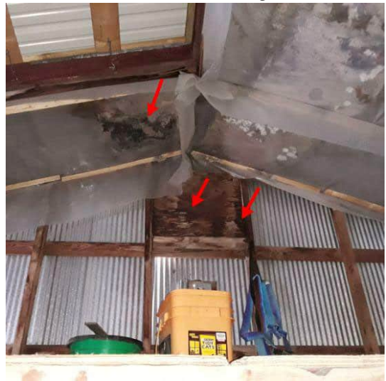
Third Floor West ceiling and wall
