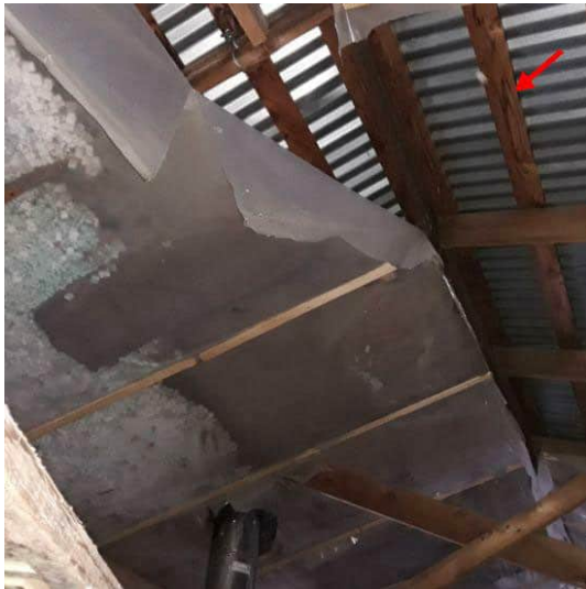
Third Floor West ceiling
