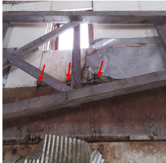
First Floor East Wall B
