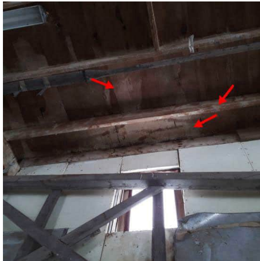
First Floor East Ceiling
