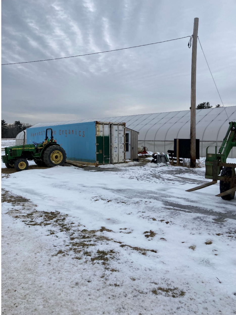
5. View of building site from the southeast corner of the "Farmstead Area" looking southwest.
