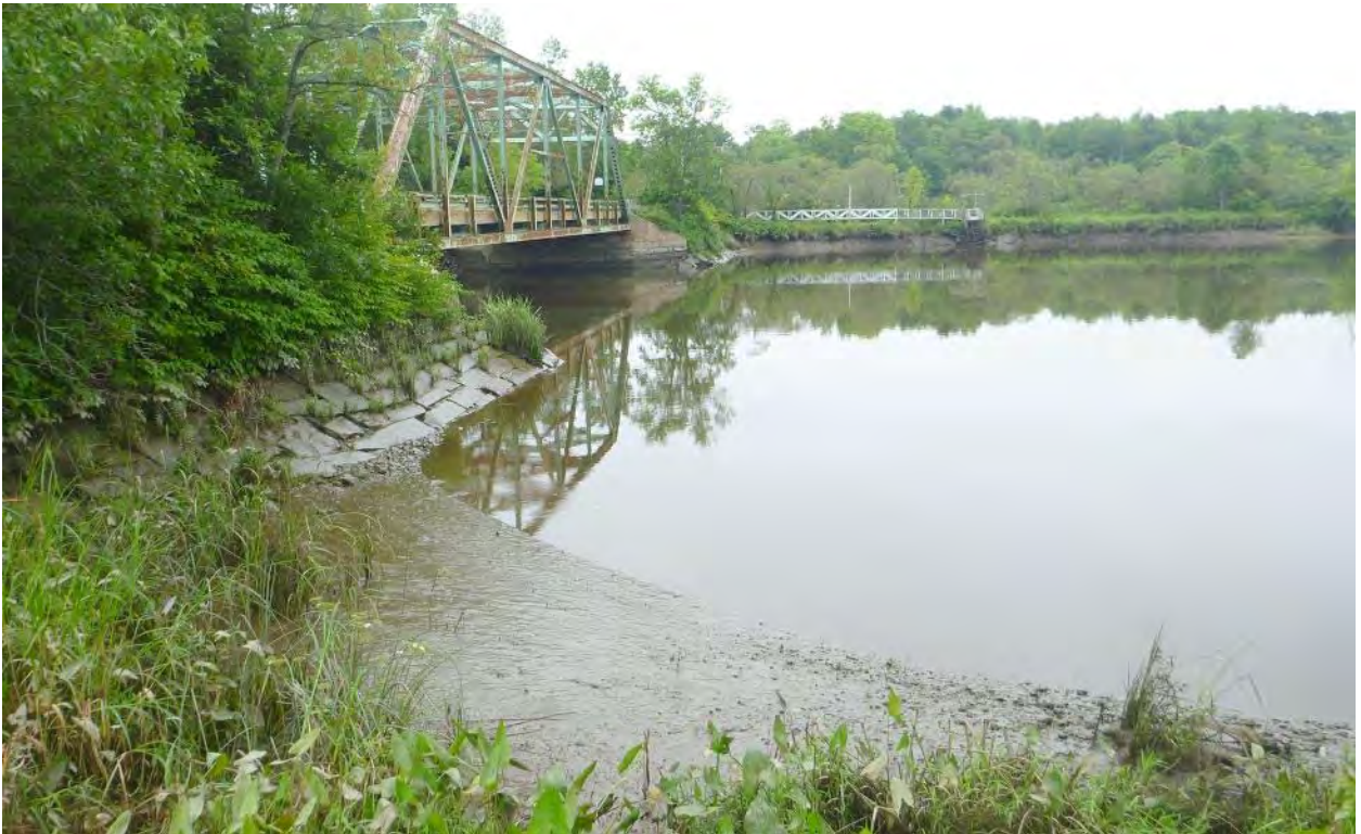
Looking east across Cathance River at proposed stone armored stabilization area. Low Tide 9:47am [Photo Time – Date: 8:10am – 8/13/18; Flow Tide]
