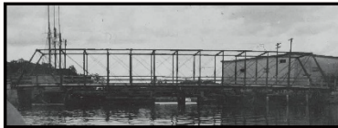
Cast Iron Bridge, 1930 144 feet long, it was a Whipple "trapezoidal truss" bridge.
