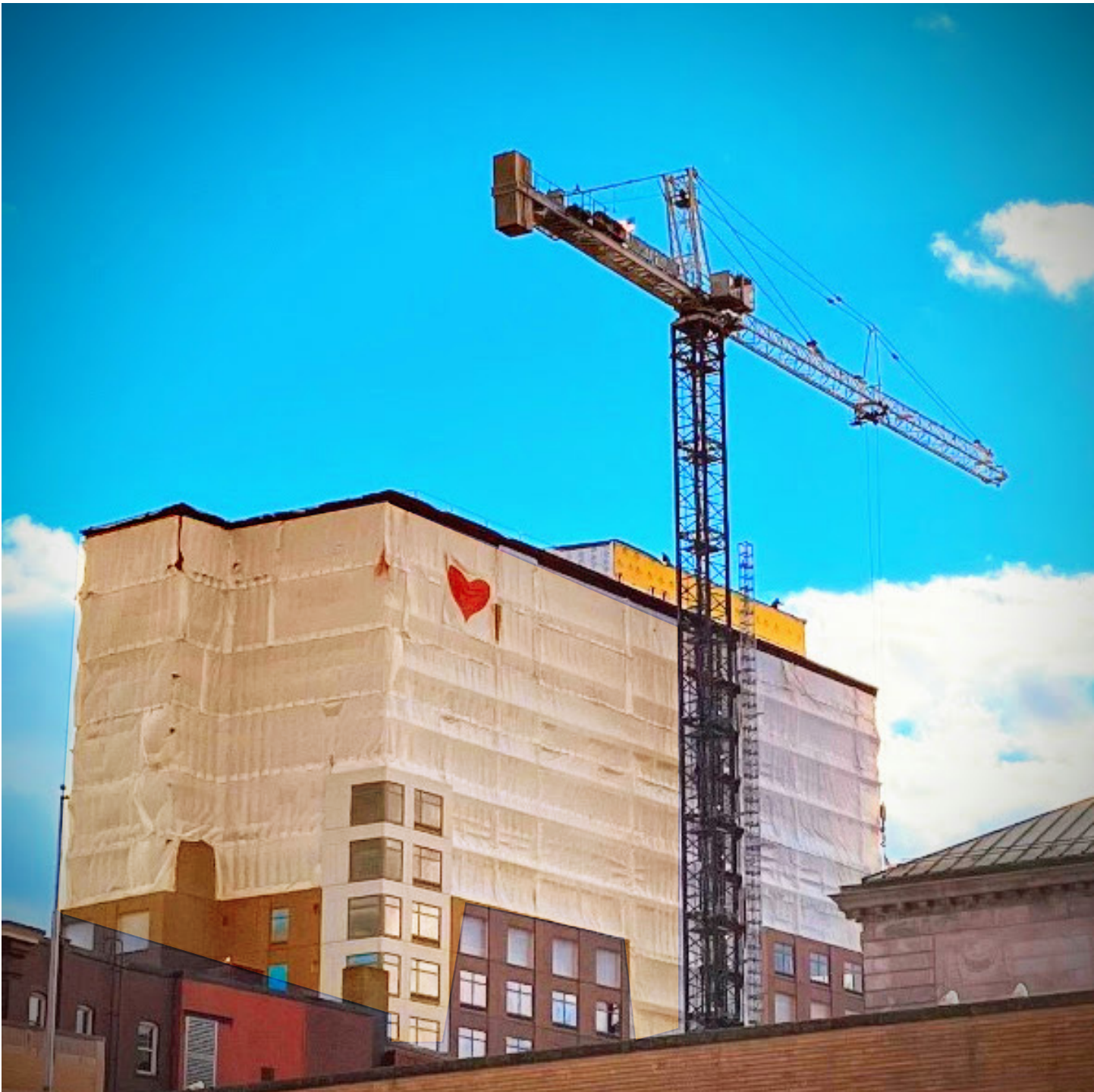
201 Federal St., Portland, ME an Acorn Engineering project
