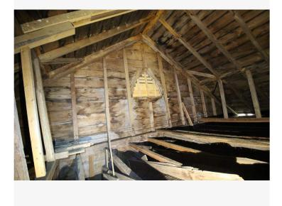
Bent 6 rear gable wall. Bent 6 is studded and contains the framing that once supported a triangular window similar to the one in the front wall of the tower.
