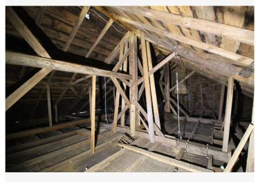
Bent 4 truss. The bent 4 bottom chord has suffered extensive water damage, and has been stabilized with 2x10 KD sisters and additional KD struts that sandwich both the upper chords and bottom chord. There are two additional chains that hang from the principal rafters and support the bottom chord between the king post and the eave plate.
