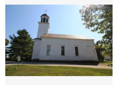
North eave elevation. This photo shows how the rear wall of the tower is stepped back from the main front gable wall.
