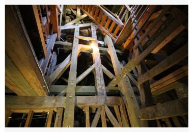
Looking west and up into the trusses. The hewn king post can be seen at the center of all this framing. A lot of framing has been added and primarily attached without joinery and with through bolts. It appears that the builder was attempting to load the tower onto the narthex wall, which isn't a bad idea.
