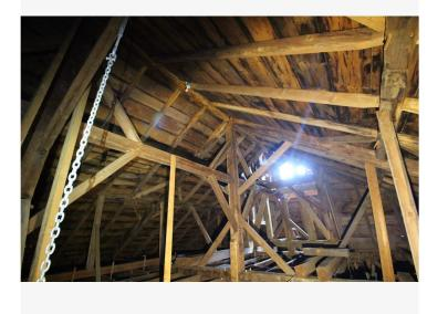
Bent 3 truss from behind, looking east. The trusses are well braced.
