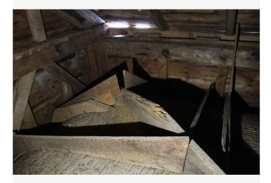
The ceiling cove is framed by 1x12 ribs with the profile of the cove cut into them.
