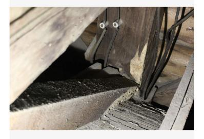
Bent 5, south post. The south post is moldy at the intersection with the ascending brace. Both the brace and post will need to be repaired.
