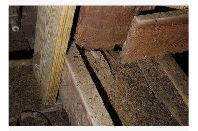
Bent 4 truss. There is extensive rot inside the king post mortise.
