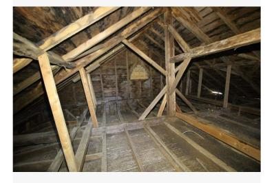
Bent 5 truss. The second set of struts is farther out on the tie beam, and meet the rafter under the intersection with the principal purlin. They do not appear to be original to the truss construction.
