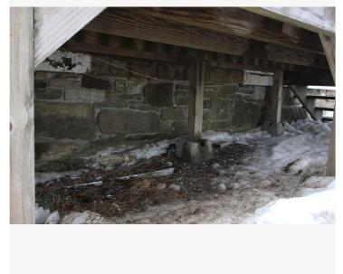
This stone wall is unusual for a building of this age. It is more typical for the foundation to have a fieldstone foundation below grade and capped with granite capstones. It is common for a dry-laid foundation to be infilled with mortar, but it is uncommon for the stones to vary so widely in size.
