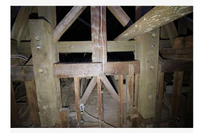
These large vertical bolsters and through bolts take the place of timber frame joinery. They are working for now. Through-bolts should be checked periodically for tightness.
