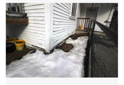
Behind the ramp, the grade pitches toward the building and directs rainwater under the building. Water and snow get trapped in the gully between the ramp and building.
