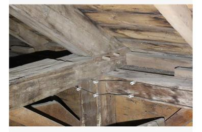
Bent 4 truss. South rafter heel is also tight. Bent 4 is referenced towards the rear.
