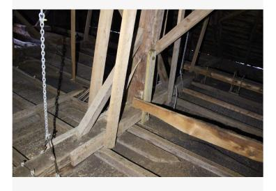
Bent 4 truss. The bottom chord, like the rest of the attic, is covered in bat guano
