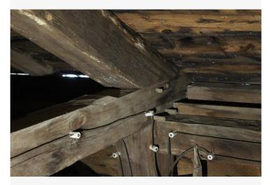
The joinery at the heel of the bent 5 principal rafter is also remarkably tight. However, the body of the rafter itself is showing signs of mold.
