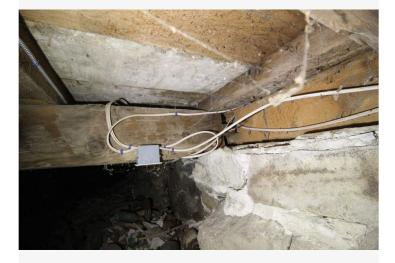
The large floor girts do not join to the new south eave sill. The sill is quite undersized and do not appear to have ever engaged the joinery.
