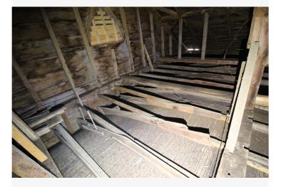
The bay in front of bent 6 gives a good view of the framing that supports the coved ceiling.
