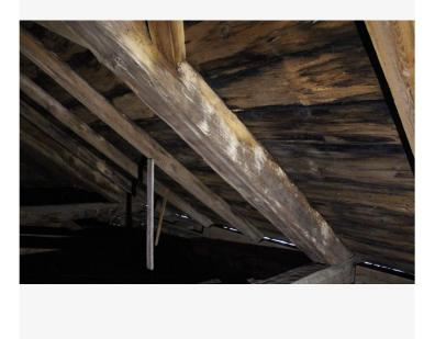
Bent 5 south rafter. The Bent 5 rafter shows significant water staining.
