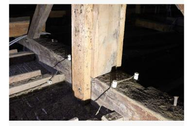
Bent 3, the bottom of the king post, where it intersects the bottom chord, is gusseted. A stirrup strap would provide more support.
