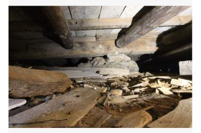
The longitudinal summer beams are picked up on stone piers, which lends the floor system significant stability.
