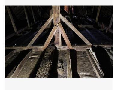
Bent 5 truss. The bottom chord is also rotted directly beneath the king post. Two gussets have been added to stabilize the bottom chord, but this is not a long-lasting repair.
