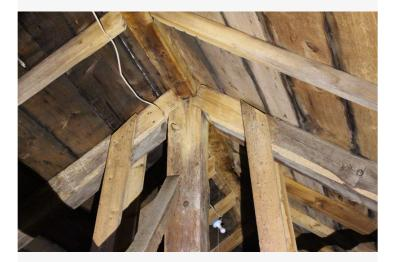
Bent 4 king post head. The joinery at the top of the king post is tight.
