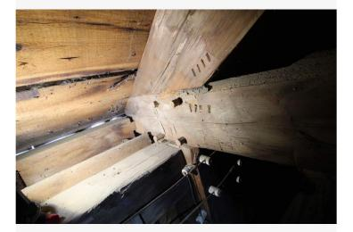
Bent 3, south end of bottom chord. The marriage marks on this and other trusses indicate that the bents were originally numbered from back to front.
