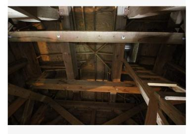
The belfry posts are supported on a stack of timbers that crisscross the tower plates. The long additional posts are visible at the very top of the frame, attached to two of the belfry bed timbers with angle iron
