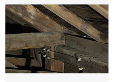
The principal rafter is connected to the bottom chord with a mortise and tenon, which is double-pinned.
