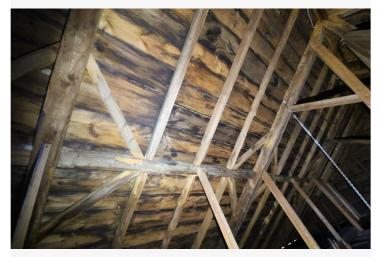
The Bowdoinham Town Hall has a very strong roof system. It is composed of principal rafters connected by horizontal principal purlins and braces. Common rafters support the roof between the bents; they start at a flying purlin in the eave cornice, cross the principal purlin, and meet at a ridge purlin in the peak.
