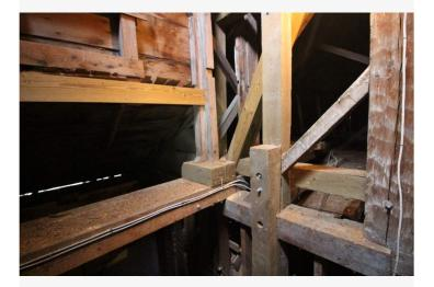
South tower bed timber. The rear corner stud of the plinth frame is landing on the bed timbers here, the rear tower post is behind the Bent 2 truss.
