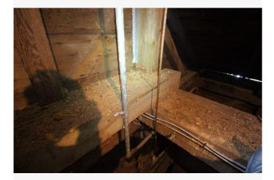
Front tower sleepers cross bed timbers and support SE tower post. The post has been severed and is secured to the sleepers with angle iron and lag screws.
