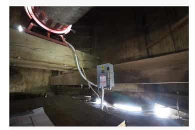
The siren is supported on bed timbers that span the belfry interior and are attached to the belfry posts.
