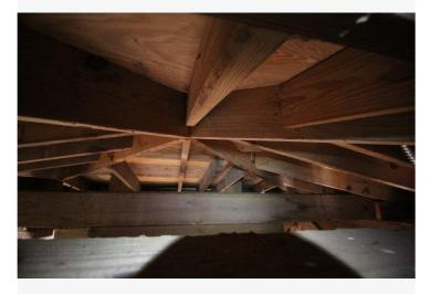
The tower roof is a new addition from the 1990s, and is a conventionally-framed hip roof.
