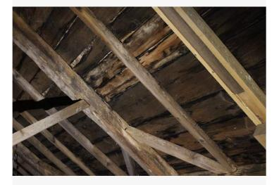
The sheathing shows extensive damage and water staining, not all of it recent.
