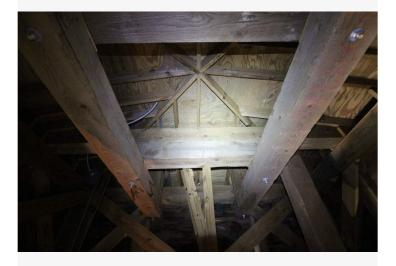
Belfry crab, looking south. The lower two belfry bed timbers cross beneath the plate, and the upper bed timbers criss above the plate. A bolster fills a void the thickness of the plate. The bed timbers are through-bolted together.
