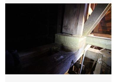
NW tower post, short blocks. The post is relieved on the rear face so that part of the bottom of the post foot is not in contact with the blocks.
