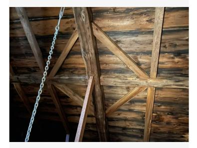
Ascending and descending wind braces in the roof plane lend the roof system extra stability.
