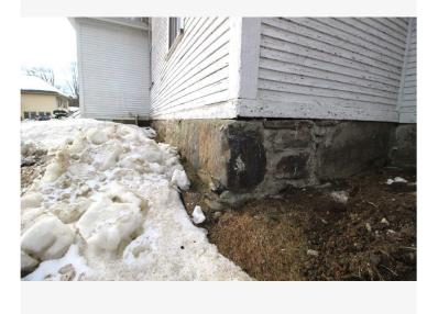
This capstone is proud of the wall plane. Water that lands on this corner can be redirected into the building, rotting the framing from the foundation up.
