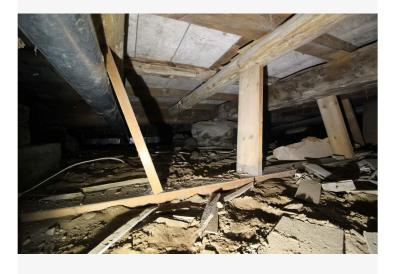
The log joists are supported at the midspan by little 2x8 kickstands. These stand on long 2x8s laid in the dirt, and are a temporary repair.
