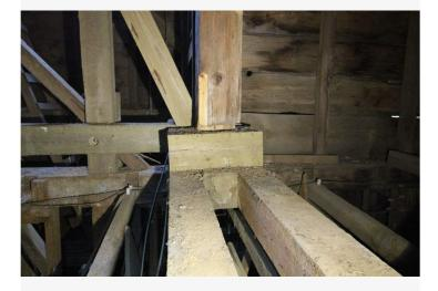
South bed timbers, blocks and SW tower post. These tripled bed timbers appear to be cut from completely new material. The center timber is not original.
