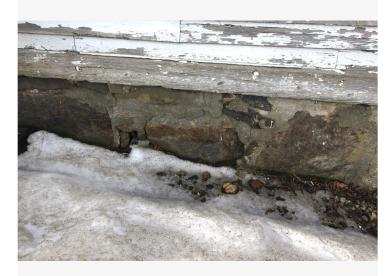
The infill mortar work varies in neatness and skill, and appears to have been applied in multiple generations.
