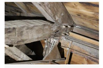
Bent 3, principal rafter and bottom chord. The north end of the bottom chord has a hole in the end that will require a face fix or other repair. The marriage marks indicate that the bents were originally numbered from rear to front.
