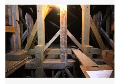
Bent 2, rear tower wall. Two additional 8x8 posts have been installed on either side of the king post.
