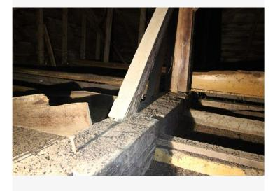
Bent 5 bottom chord and king post connection. The bottom chord has separated from the king post and the descending braces. There is rot in the king post mortise.
