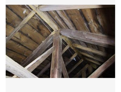
Bent 3 king post. The joinery between the principal rafters and the head of the king post is tight.
