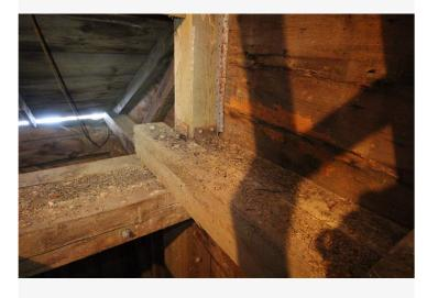
At Bent 1, the south gable, two sleeper timbers cross the tower bed timbers.
