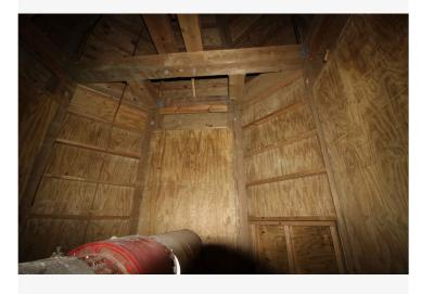
Belfry interior. The belfry walls are conventionally framed out of 2x4s and 2x6s, and sheathed in plywood.
