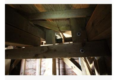
Belfry crab and post, north tower plate. In the background, the additional Bent 2 posts can be seen crossing the upper belfry bed timber.
