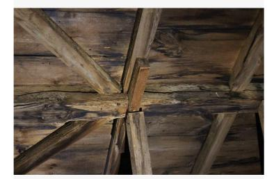
This principal purlin has been severed at the first common rafter, and will need to be replaced.
