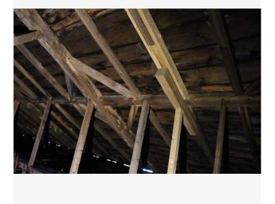
Bent 5 rafter shows significant water damage, and a common rafter in the bay behind it has rotted through and been repaired with gussets and a bolster.
