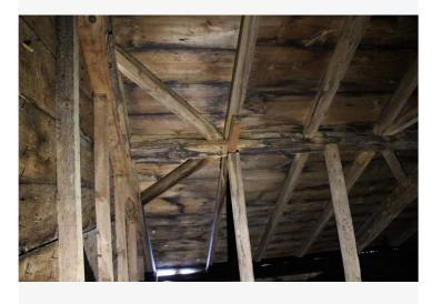
The principal purlin between bents 5 and 6 is badly rotted, and is being stabilized with a couple of struts.
