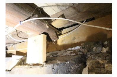
Another log joist end showing signs of rot, not connecting with the eave sill, and propped up on a rickety 2x8.
