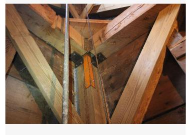
When the SE post was installed, all joinery was severed. Many of the tower girts were also replaced, and connected to the tower post with angle iron. Unfortunately, the tower posts were undersized, and there are significant gaps between the ends of the girts and the face of the tower post. These should be filled, and additional shear blocks installed.
