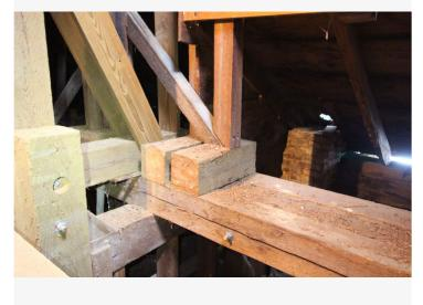
North tower bed timber and sisters. The tower beds cross from Bent 1 to bent 3 and pick up the tower posts, and other framing, like this stud and brace. The original bed timber was at 8x8 and is sandwiched between two new 8x8 sisters.
