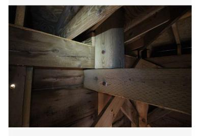
The belfry posts land on the belfry bed timbers, and are through-bolted. A section of angle iron crosses the joint on the opposite side. Everything is secured to the plates, but are the plates secured to the tower posts?
