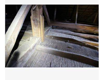
Bent 3, the bottom of the king post is gusseted on both faces at its intersection with the bottom chord.
