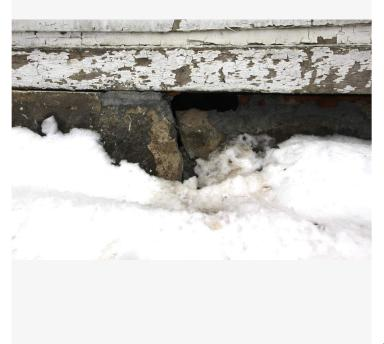
Despite mortaring attempts, this north eave foundation stone has tipped into the crawl space.
