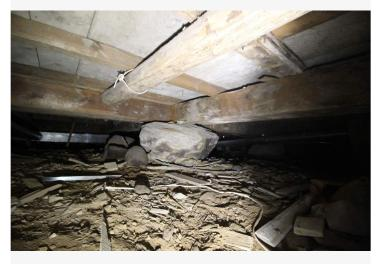
The floor is bisected longitudinally by two major summer beams. These are intersected by large floor girts aligned with the bents. large log joists intersect the summer beams and eave sills, parallel with the floor girts. The major intersections on picked up on stone piers, which has significantly contributed to the longevity of this frame.
