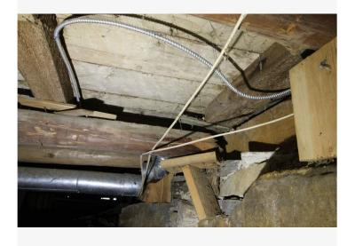
The ends of the log joists show signs of rot. They do not connect with the replacement sill.
