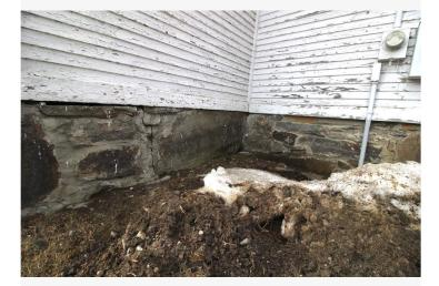
Recently, movement has been observed in the foundation. Here a long crack is visible in the mortar.
