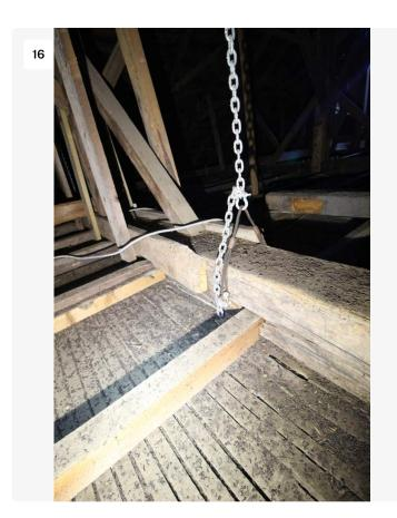
Bent 4 truss. Past the sisters, the bottom chord is picked up with a chain and cable, between the king post and the plate.
