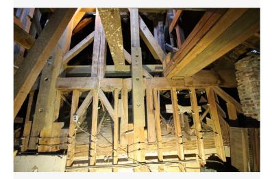
The posts land on the narthex wall. It would seem that the builder was attempting to transfer the belfry load to the narthex wall. It is unclear whether this was successful. Vertical bolsters reinforce the butt cut connections.
