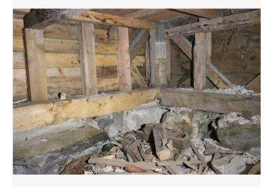
Southwest corner. A new south sill has been installed without engaging the undercarriage joinery. The new sill is about 3" narrower than the original sill.
