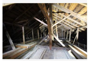
Bent 3 truss. The truss is composed of a king post (at the center of the triangle), two upper chords (or rafters), one bottom chord (or tie beam), two ascending braces (or struts), two descending braces and two additional struts farther out on the tie beam.
