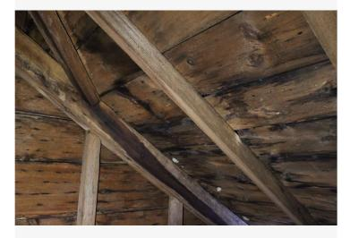
The north rafter in bent 6 also shows extensive water staining. We anticipate it will need to be repaired.
