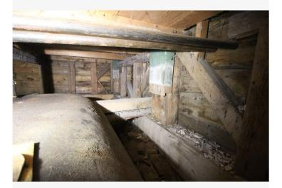
Entrance to the crawl space from the stage hatch shows wall framing below the stage. A mid-wall timber is wide and shallow, and shows the remains of former casing.
