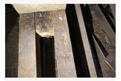
North bed timber and block. The center timber appears to be the original bed timber and has been severed and sistered.
