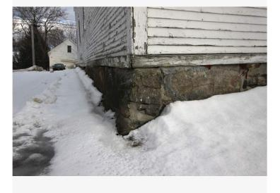
Northwest foundation corner. This section has moved dramatically, and shows multiple repair attempts. The footer is not adequate to withstand annual freeze-thaw cycling.
