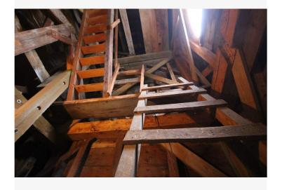
Looking north and up into the tower. The walls have been extensively braced with additional 2x8 kiln-dried lumber.
