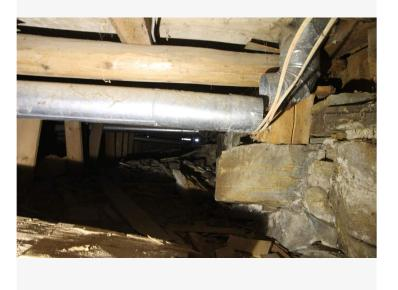
This duct work is disconnected. Ducts will need to be serviced.
