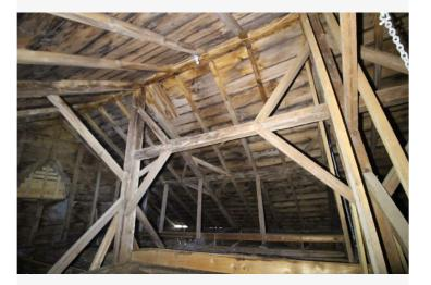
Bent 4 to Bent 5 trusses. The trusses are connected by a longitudinal girt, a pair of ascending braces and a pair of descending braces.
