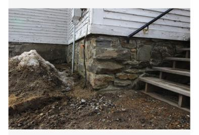
The foundation has received many generations of repair. Above ground, it is mortared, with stones of widely varying size.
