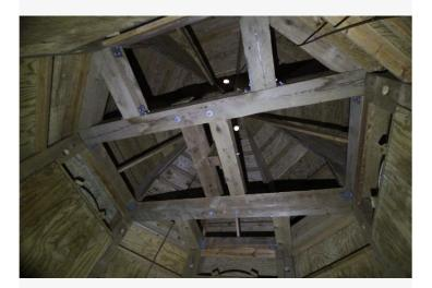
Belfry dome crab. The crab that supports the dome has been rebuilt out of new 8x8s, and bolted together. It is likely that this arrangement of timbers mimics the original timber-framed crab design.
