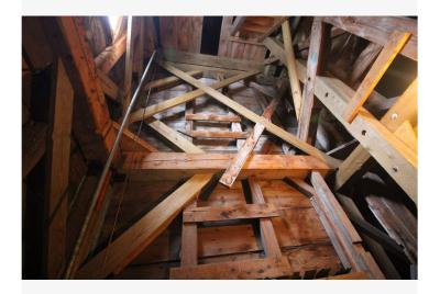
Looking south and up into the tower. The tower contains both original bracing and later stabilization bracing made from long pieces of dimensional kiln-dried lumber.
