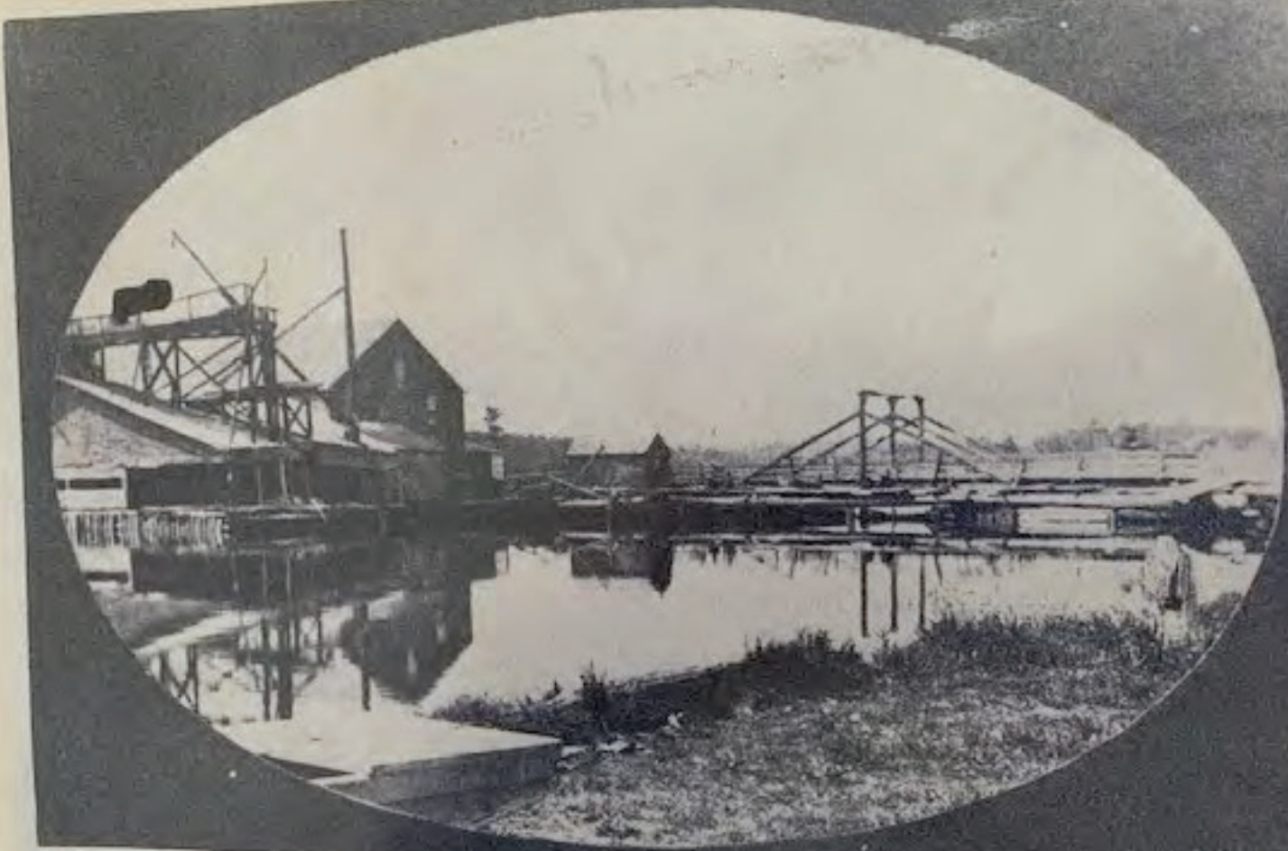
This early view of Kendall's plaster-fertilizer mills was taken when the bridge over the Cathance was a wooden, king-post span. The mill, on Bowdoinham's Brooklyn shore, burned about 1900.
