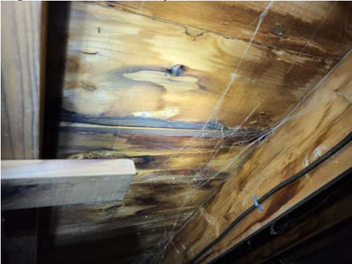
Wood is weathered in some areas, with minor signs of mold growth (black streaks)
