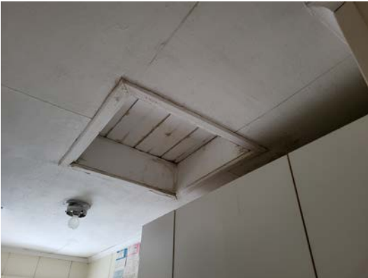
Access to Attic in Hallway
