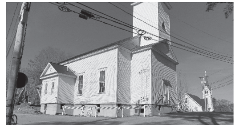
Resting on New Foundation
