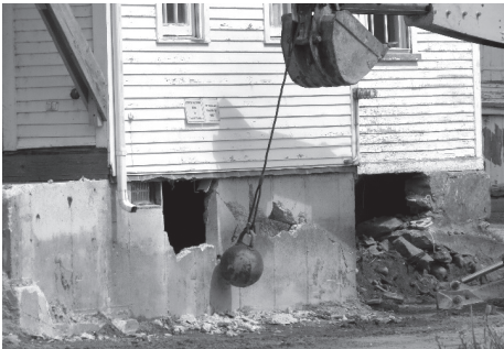
Removing the old foundation
